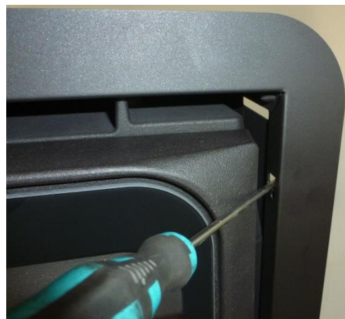
Figure No.13 - How to bend the tabs
